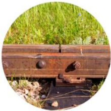
Insulation joint fishplate damage
